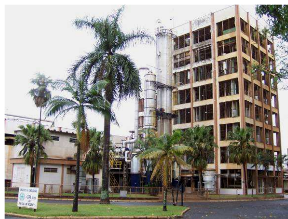
Figure 8: Sugarcane bioethanol plant (Brazil) [A]
