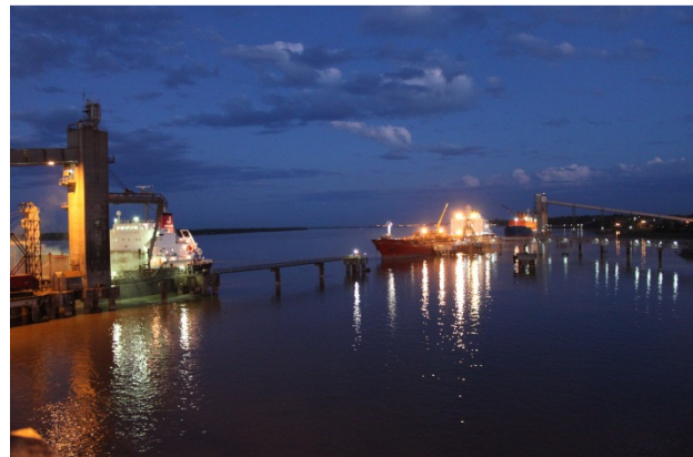
Harbour facilities for loading soybean into ships at the Paraná River at Dreyfus in Lagos
