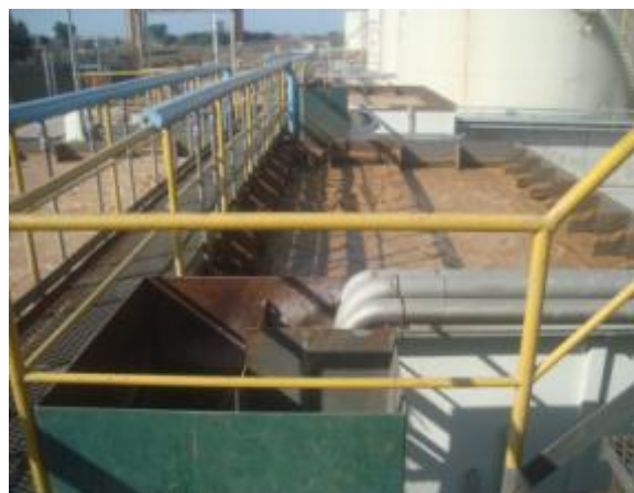
Picture 12 Activated sludge biological treatment plant.
