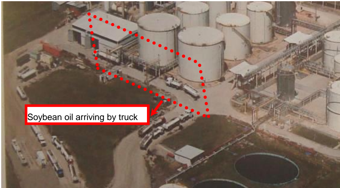
Picture 1 Feedstock Discharge
